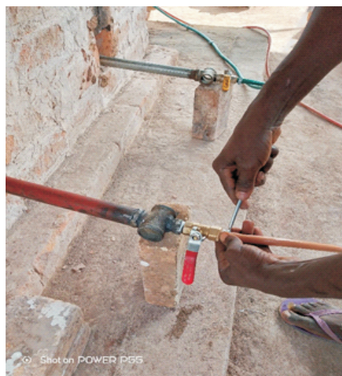
Fig. 7: Inserting the fabricated burners in a kiln
